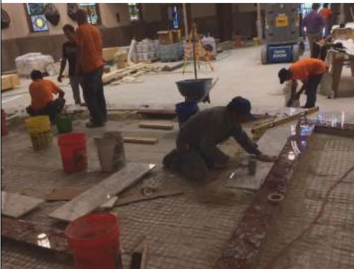
Marble tile being installed in the Sanctuary.
